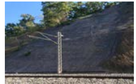
Reconstruction of slope using a flatter gradient, high strength rock and armoured with concrete.
