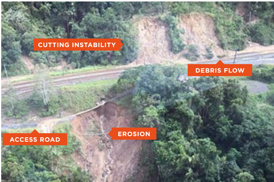
Geotechnical failures on Black Mountain due to TC Debbie
