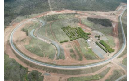
Wiggins Island Rail Loop
